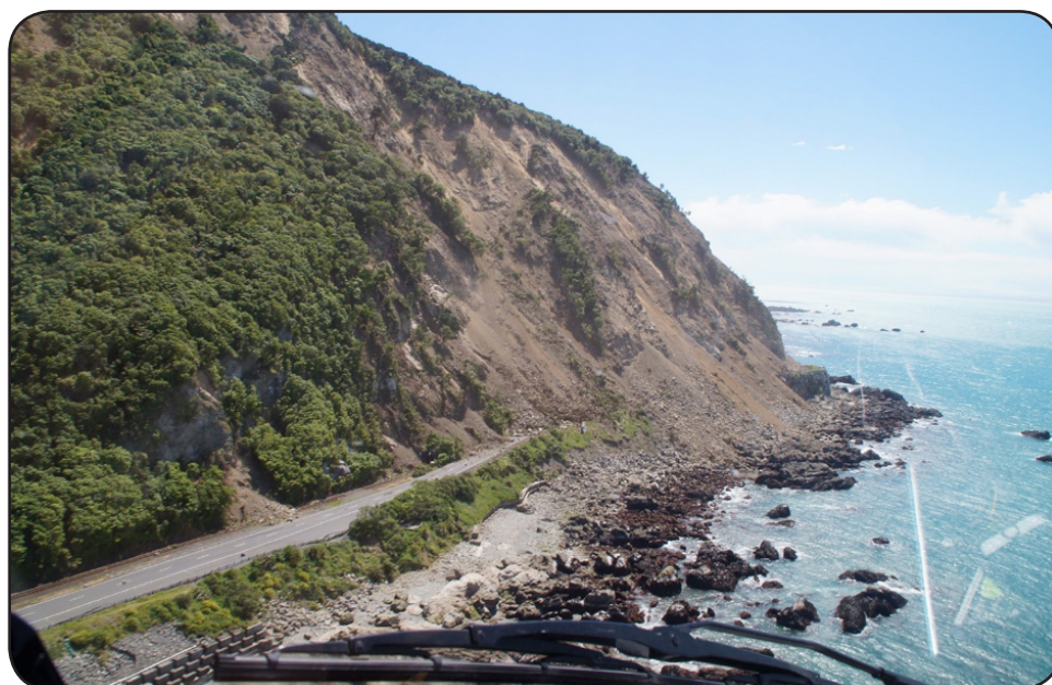
Figure 4 Landslides showing damage to the infrastructure – both road and railway
